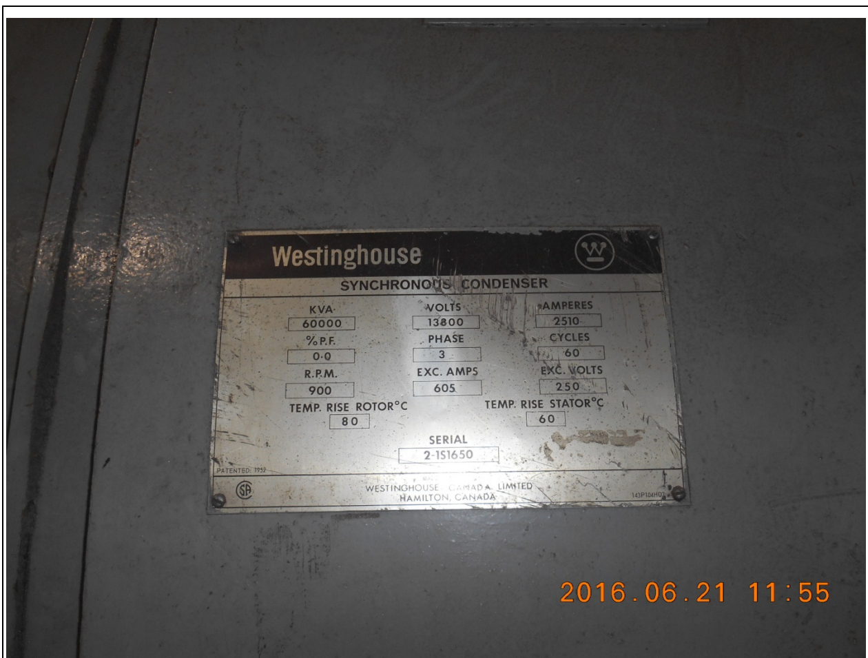
Fig. 1: Westinghouse 60MVA Synchronous Condenser
