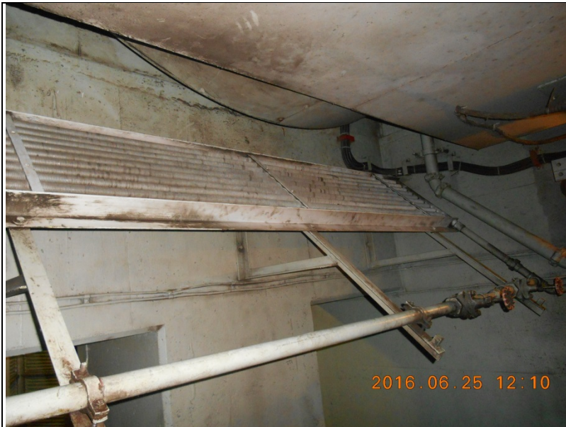
Fig. 28: Oil Cooler Condition - Typical
