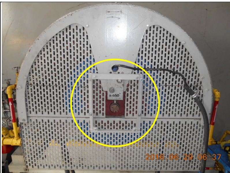
Fig. 32: CRE Guard/Cover installed
