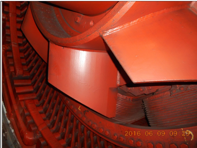
Fig. 5: Stator end turn and coil extension condition
