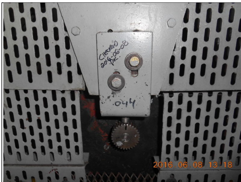
Fig. 18: Speed probe gap
