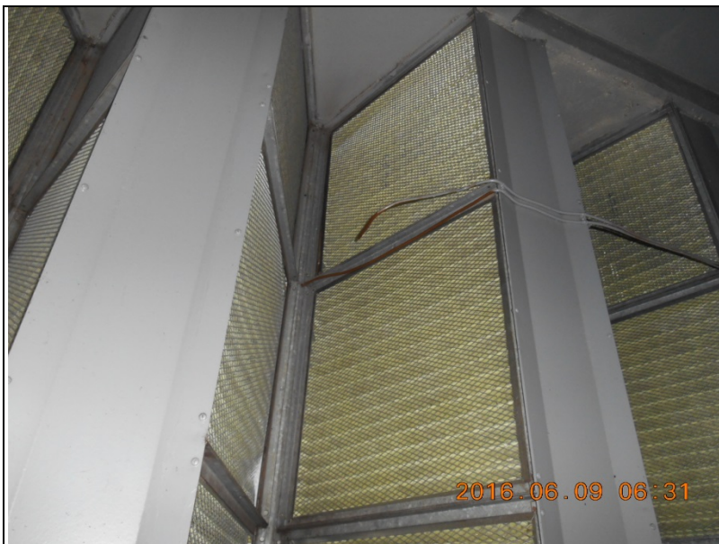
Fig. 26: Air filters
