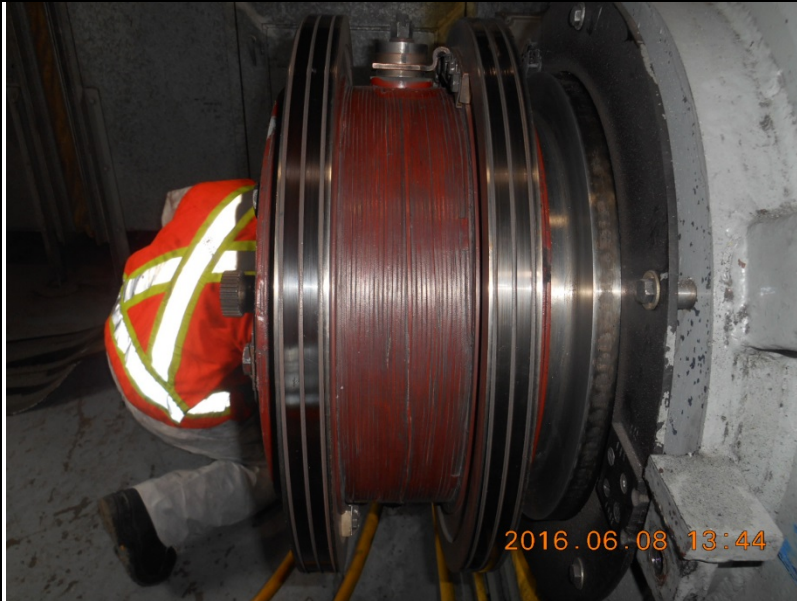
Fig. 16: Collector Rings
