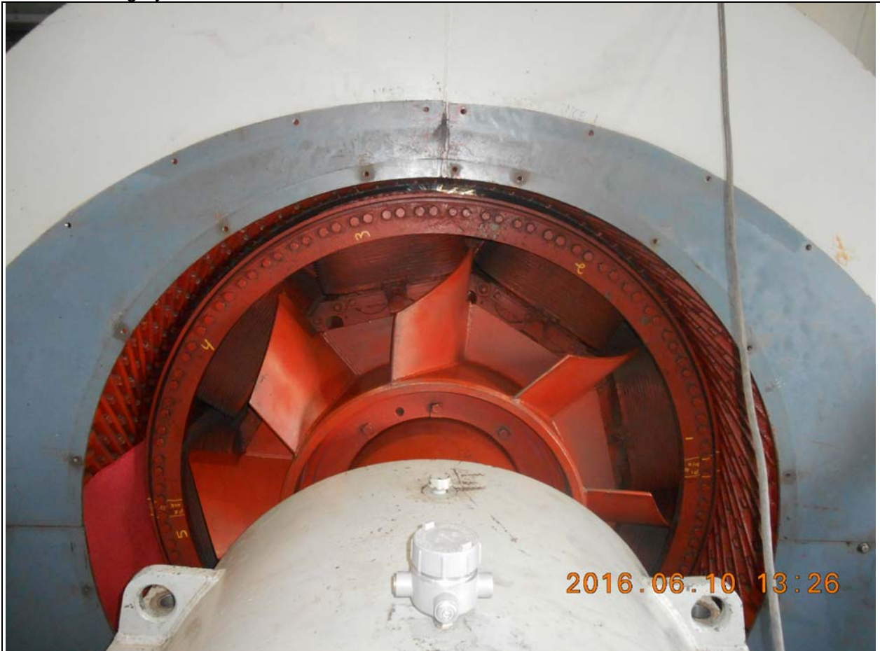
Fig. 2: Overview of Non-Collector End - Light Dirt on Stator Winding End Turns and Rotor Poles
