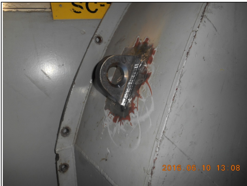
Fig. 27: New lifting lug installed
