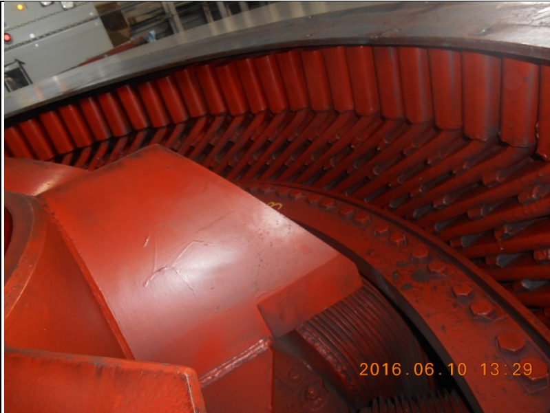
Fig. 6: Stator end turn and coil extension condition
