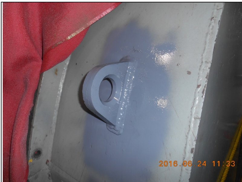
Fig. 30: New lifting lug installed on SC2 NCRE End-Bell
